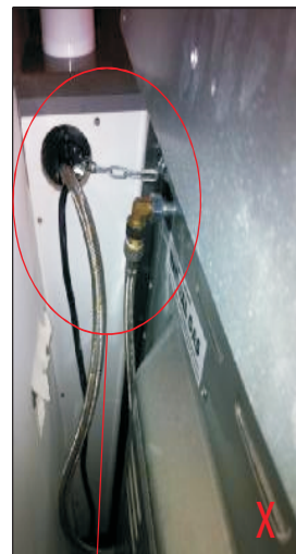
Hole in cabinet too large, Allowing the upright oven to tilt forward
