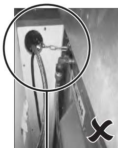
Hole in cabinet too large, allowing the upright oven to tilt forward
