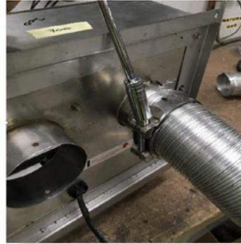
Slide flue onto connection spigot fully. Tighten clamp fully.
