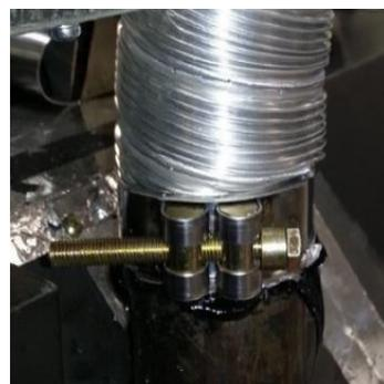
Slide flue onto connection spigot fully.
