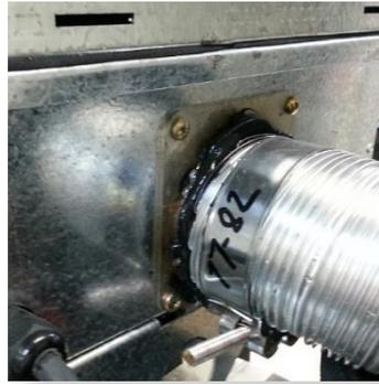
Slide flue onto connection spigot fully.
