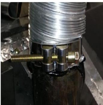
Repeat for air intake flue connection.
