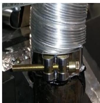
Slide flue onto connection spigot fully.
