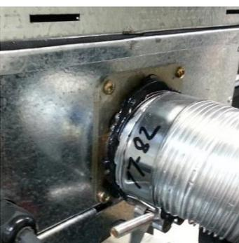
Slide flue onto connection spigot fully.
