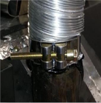
Repeat for air intake flue connection.
