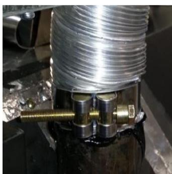
Slide flue onto connection spigot fully.
