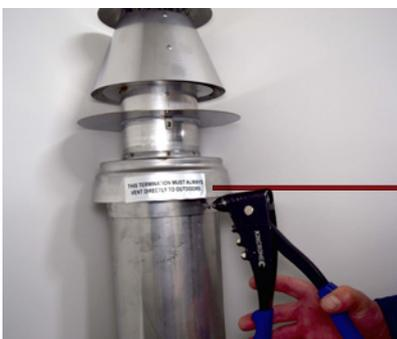
Screw or rivet in 3 places to hold in place.
